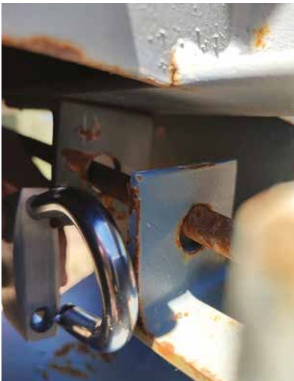
Figure 6: Capoura case, the gate was breached and the peg probably moved slightly, so the lock could not fit in both points (holes) and then locked. Michael Zacharias©Forestry Department Archive.
