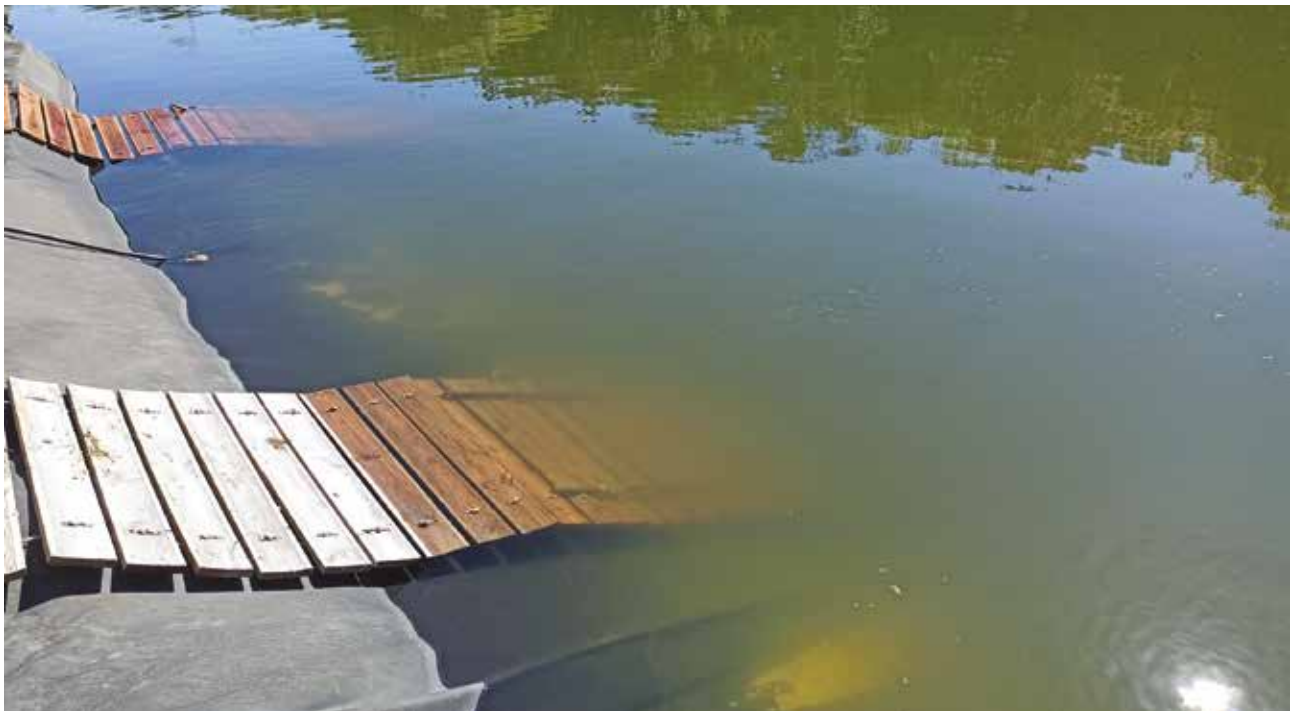
Figure 10: Traction enhancement device, stabilized in a tank with sloping walls. LIFE Bonelli eastMed©UoC-NHMC Archive.
