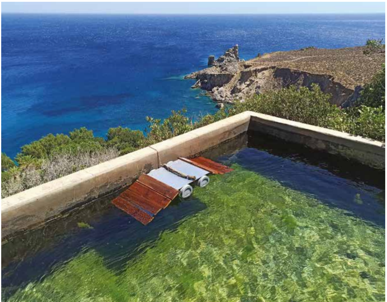
Figure 5: Floating arrangement for vertical wall tanks. LIFE Bonelli eastMed©UoC-NHMC Archive.
