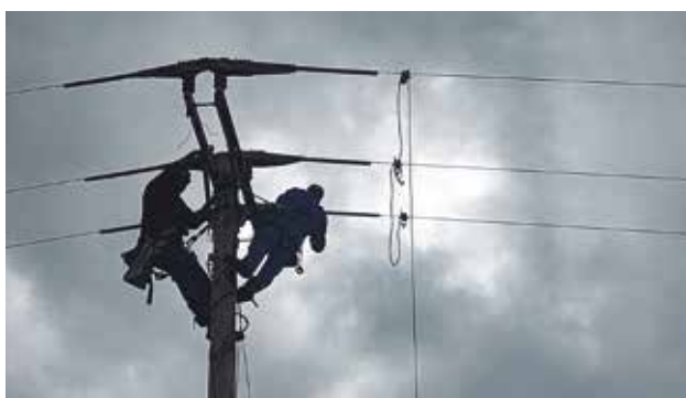
Figure 12: Example of placing covers on a straight crossarm pole with pin-types insulators in Crete (source: HEDNO - Stamatis Tomaras).
