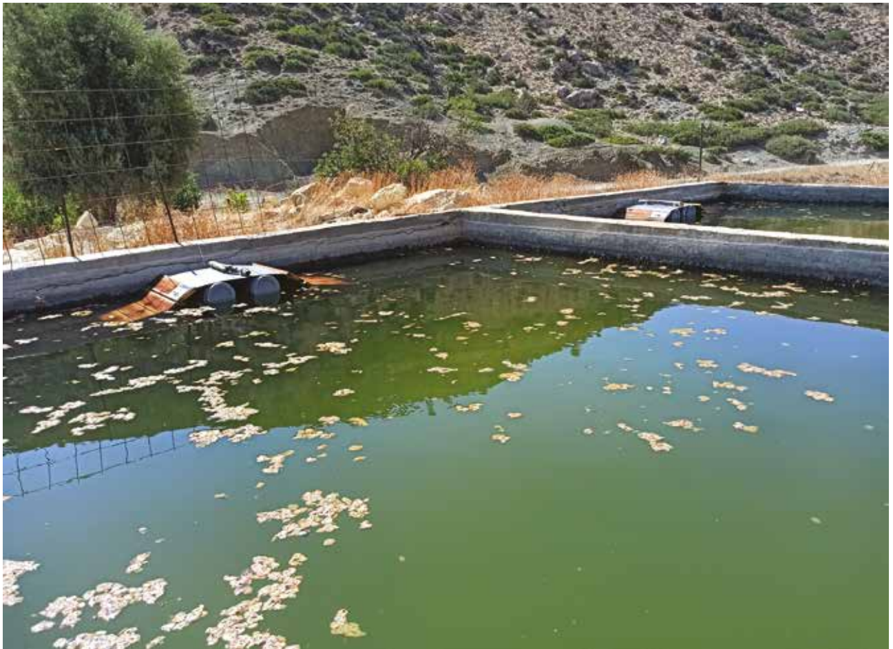
Figure 11: Model of an escape arrangement in concrete vertical wall tanks, in the framework of the LIFE Bonelli eastMed project. ©UoC-NHMC Archive.
