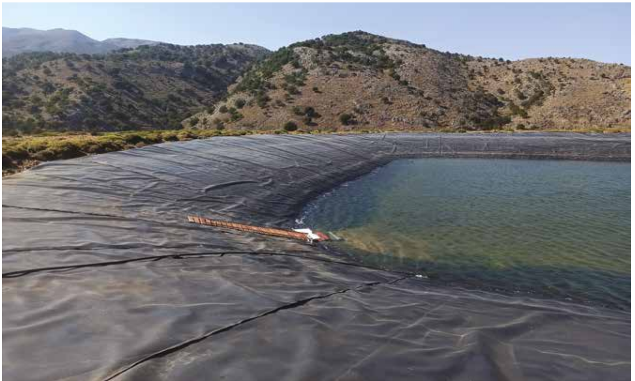
Figure 9: Traction enhancement device, stabilized in a tank with sloping walls. LIFE Bonelli eastMed©UoC-NHMC Archive.
