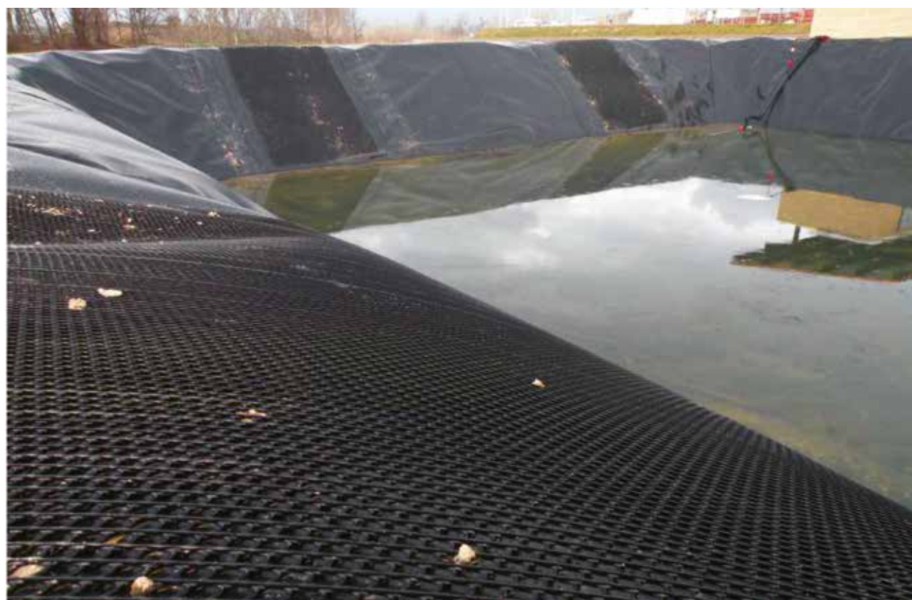
Figure 8: Heat-sealed mesh membrane. Source: NUMA Industrial S.A.
