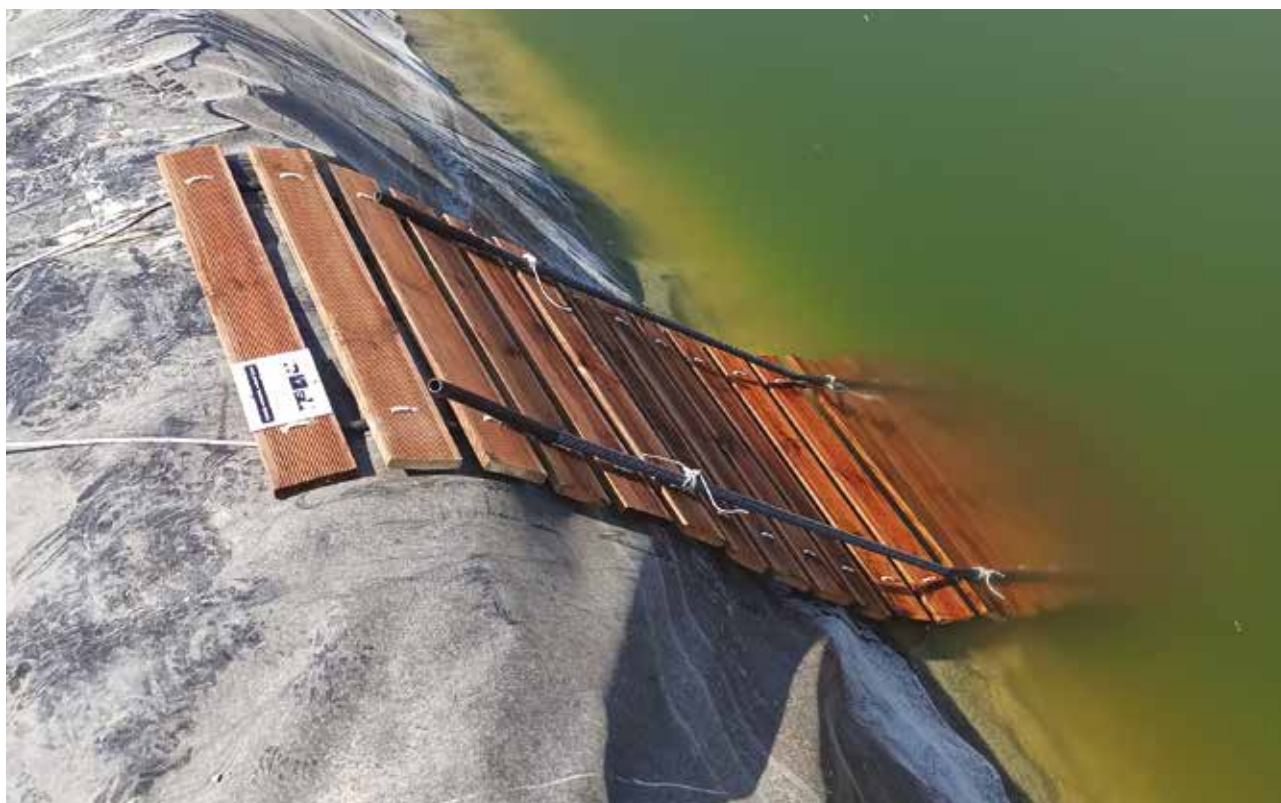
Figure 15: Correct installation of a fixed escape device. LIFE Bonelli eastMed©UoC-NHMC Archive.
